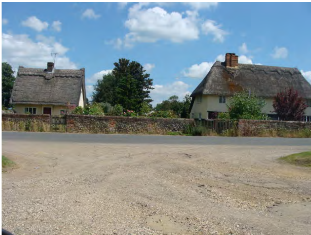
Picture 1.2 . Estate no.53 on left; estate nos. 50-52 on right of picture. This quintessential English village scene of thatched cottages with brick and flint boundary walls has remained little changed since they were originally built.
